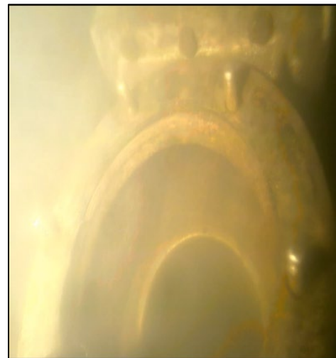
Open strainer found during dive operations.
